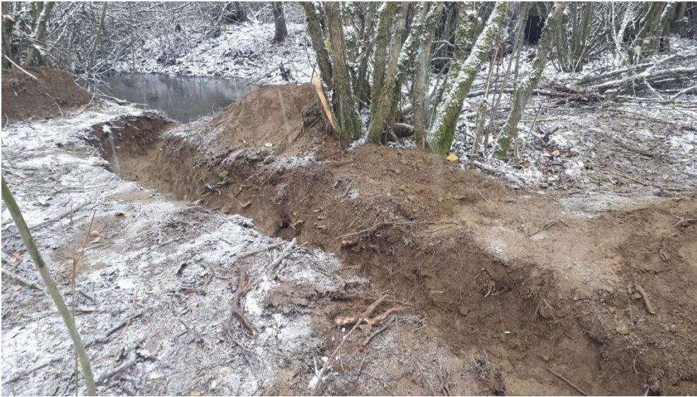
Photo 6: Bings Creek, Reach 1, immediately downstream of Site 4 a connectivity ditch was created to increase flows into an anoxic backwater pool to increase rearing habitat for fish in summer.
