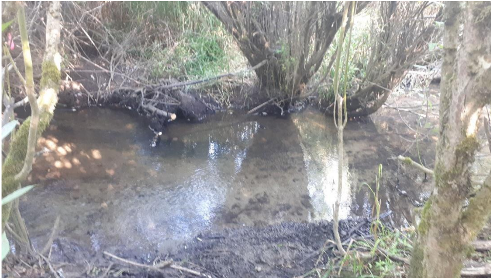
Photo 3: View looking at left downstream bank before restoration at Site 4. Habitat mainly was silt, sand, and organics.
