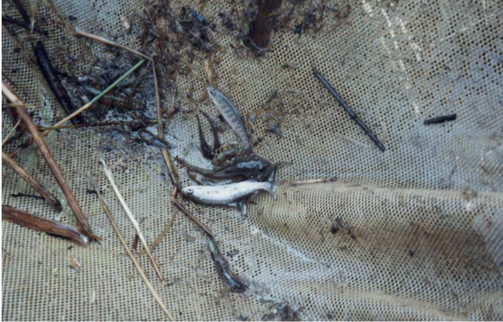
Photo 3: The fish were salvaged as the pumps were drying the sections to be excavated
